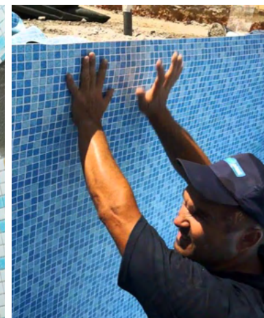
INSTALLATION OF PVC LINER
